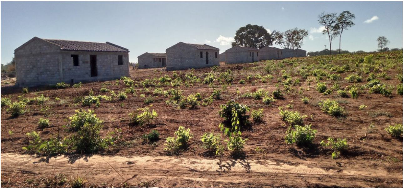
Figure 3: Mwichi community resettlement houses - approved and under construction
