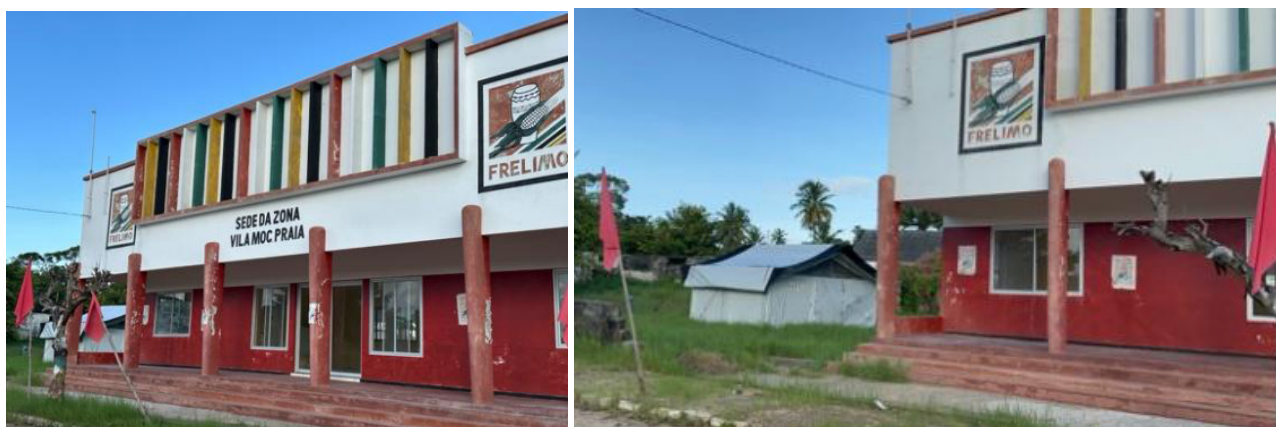
Fig. 5. Tents made available by UNOPS were installed at the headquarters of the Frelimo Party in Mocimboa da Praia
