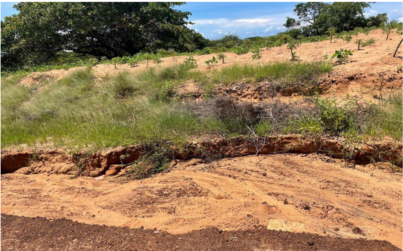
Figure 1: Access road to Thopa
